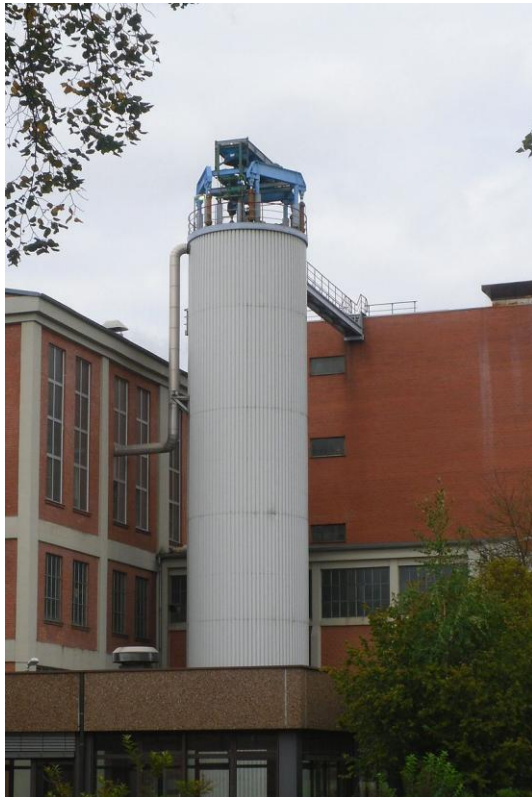
Vertical cooling crystallizer in a beet sugar factory
